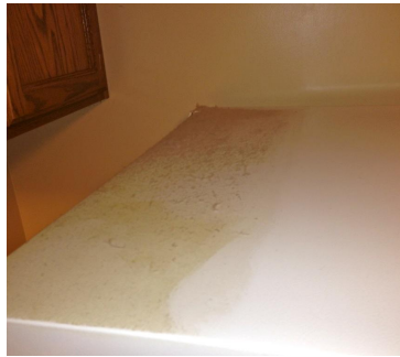
Back-half of Top of Refrigerator
